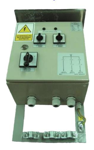
Switchgear type ZRO-1 is an electric device designed for use underground mining, in work-pits in non-explosive hazard conditions and on the ground in non-hazardous areas.
